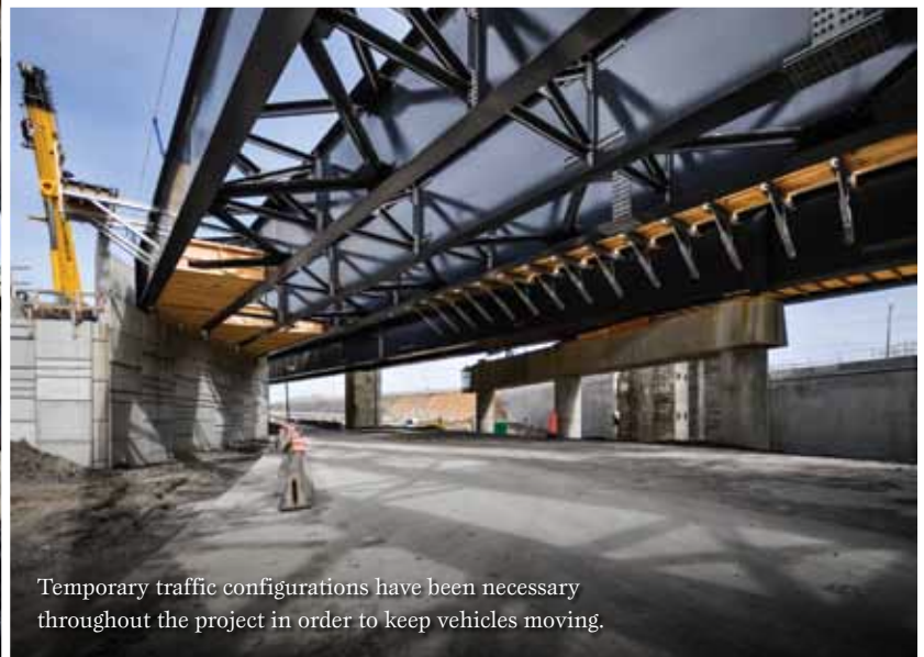
A temporary prefab launch bridge, shown here in December of 2017, was one of the innovative solutions used to reduce construction impacts on the 300,000 daily users of the interchange.
