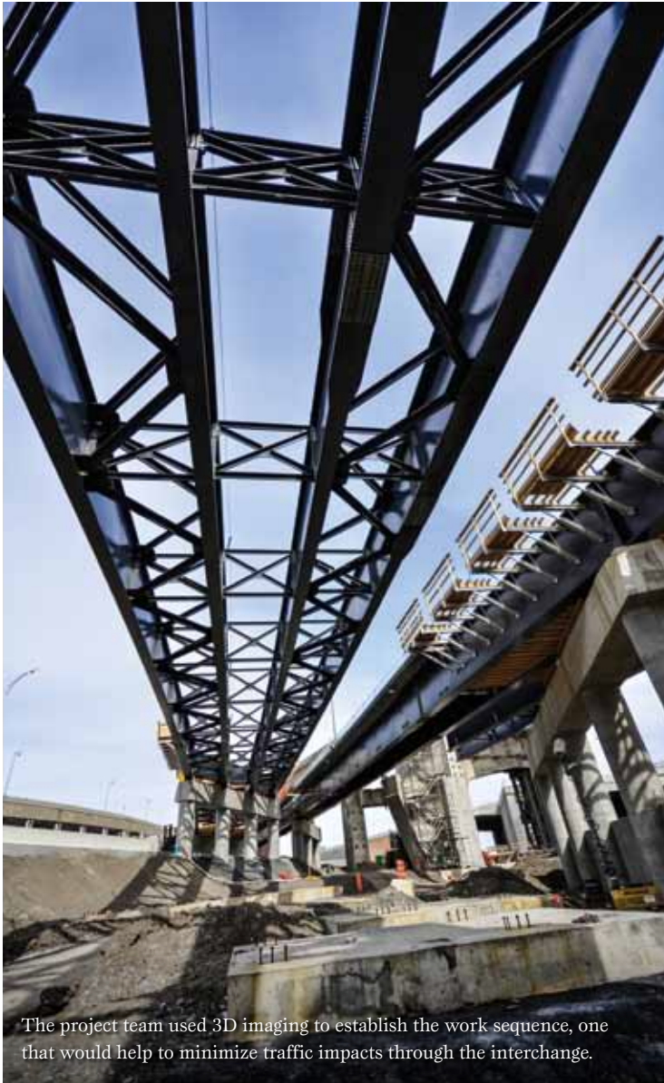
A temporary prefab launch bridge, shown here in December of 2017, was one of the innovative solutions used to reduce construction impacts on the 300,000 daily users of the interchange.
