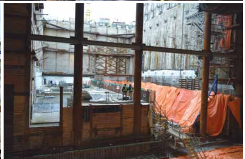
Looking west towards Mount Dennis station, preliminary work is underway to begin pouring the interior concrete walls.
