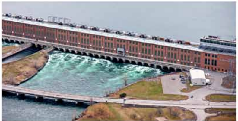
Beauharnois Generating Station, QC – Photo: Air Photo-Max
