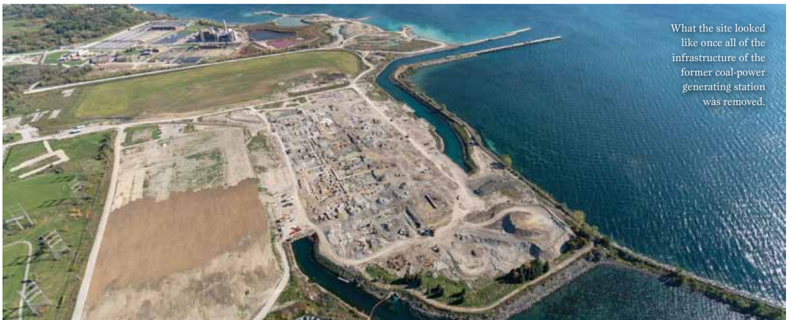
Excavators work to remove the remaining concrete from the site.
