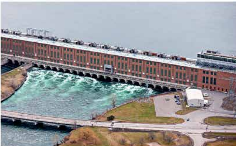
Beauharnois Generating Station, QC - Photo: Air Photo Max
