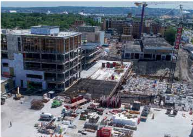
Construction site for the Quebec City University Hospital Centre - Laval University, QC
