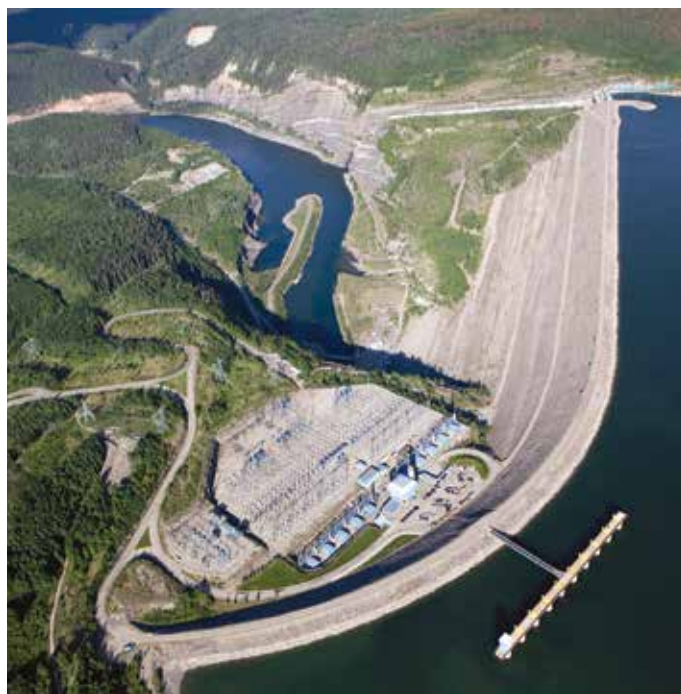
Credit: BC Hydro
