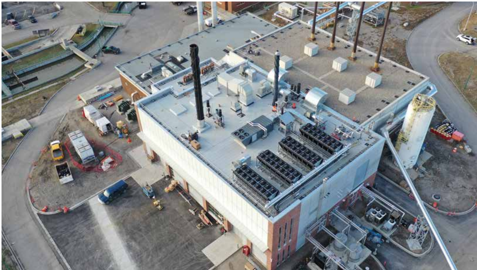
The City of Calgary's Bonnybrook Cogeneration Expansion Project takes biogas handling to the highest level: using all its biogas as the primary fuel source to meet its needs for electric power and industrial steam for its advanced treatment process.
