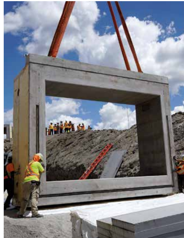
Metrolinx's Finch West LRT team took recently installed 18 concrete tunnel segments under the Highway 400 southbound on-ramp at Finch Avenue West, as part of a new multi-use tunnel.
